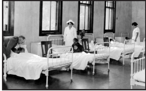
Figure 18. USIS Hospital ward, CSP 090-610
