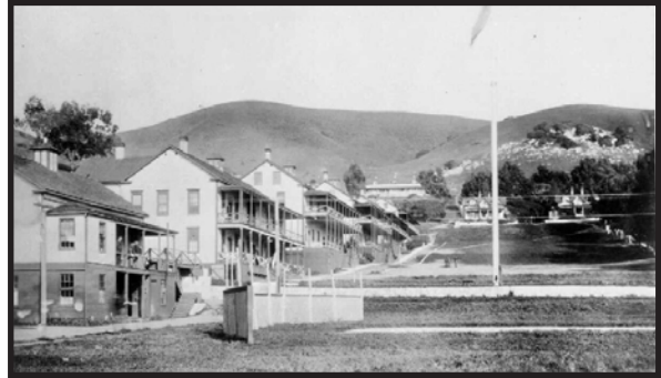
Figure 2. Camp Reynolds, CSP 090-618
