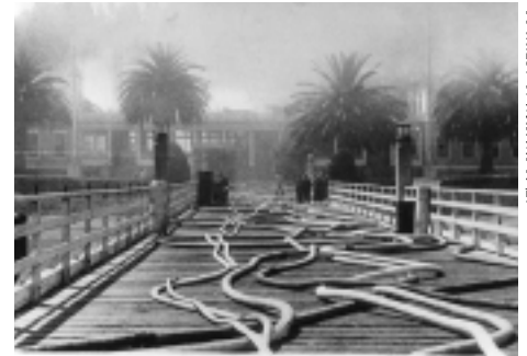
Hoses snake along the pier after the Administration Building fire, 1940.
