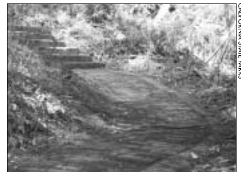
The brick pathway behind the power plant that volunteers uncovered at the Angel Island Earth Day event.
