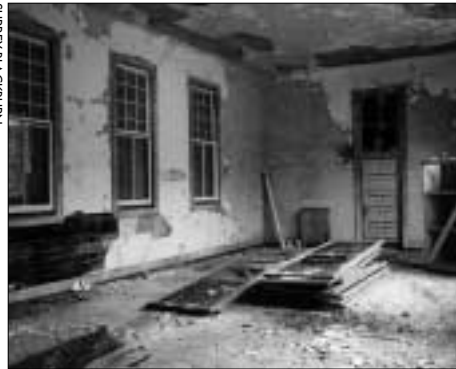
The crumbling interior of the hospital today.
